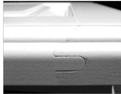
Example of door end joint separation
