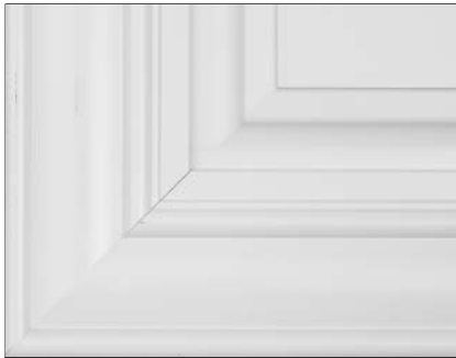
Example of door front joint separation
