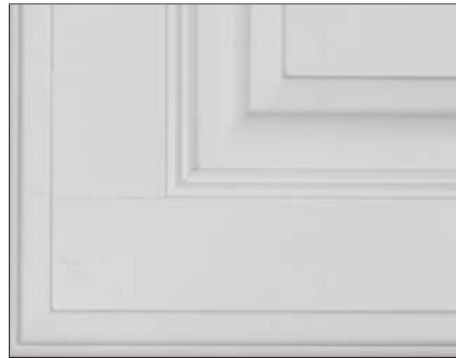
Example of door front joint separation
